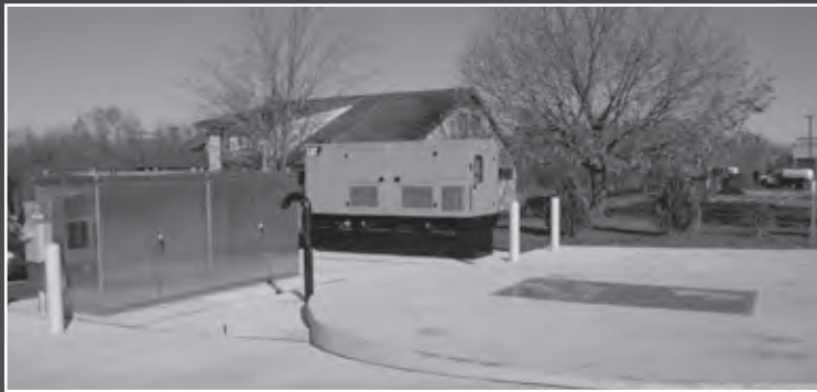
Lift Stations—New and Retro-fit Upgrades
