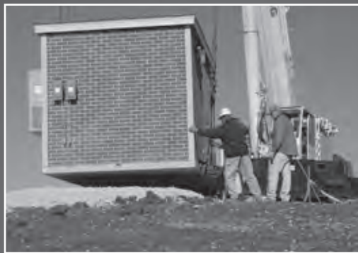
Housed Pump Systems
